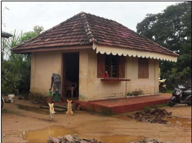
Existing Sales Center
